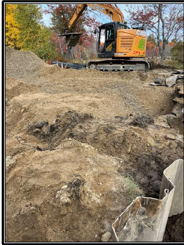
Photo 5: Compacting the roadway with the excavator bucket.
