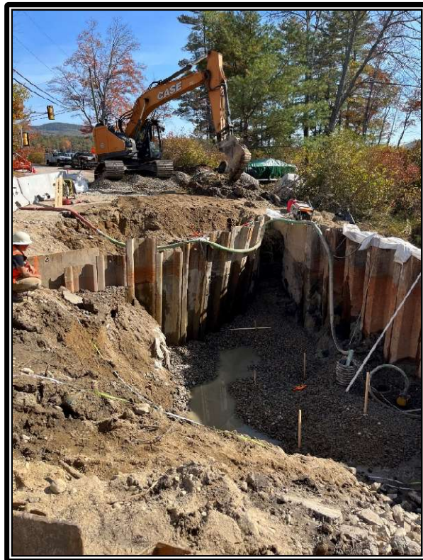
Photo 1: East wall of sheet pile is caving
