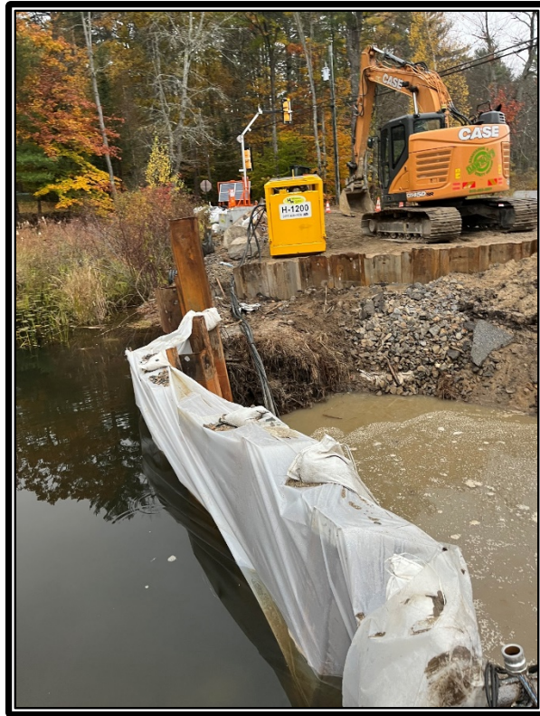
Photo 2: Water has penetrated into the excavation.
