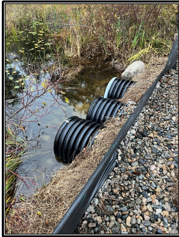
Photo 1: Water level has risen to approximately 14 inches from the bottom of the temporary bypass culvert's inlet.
