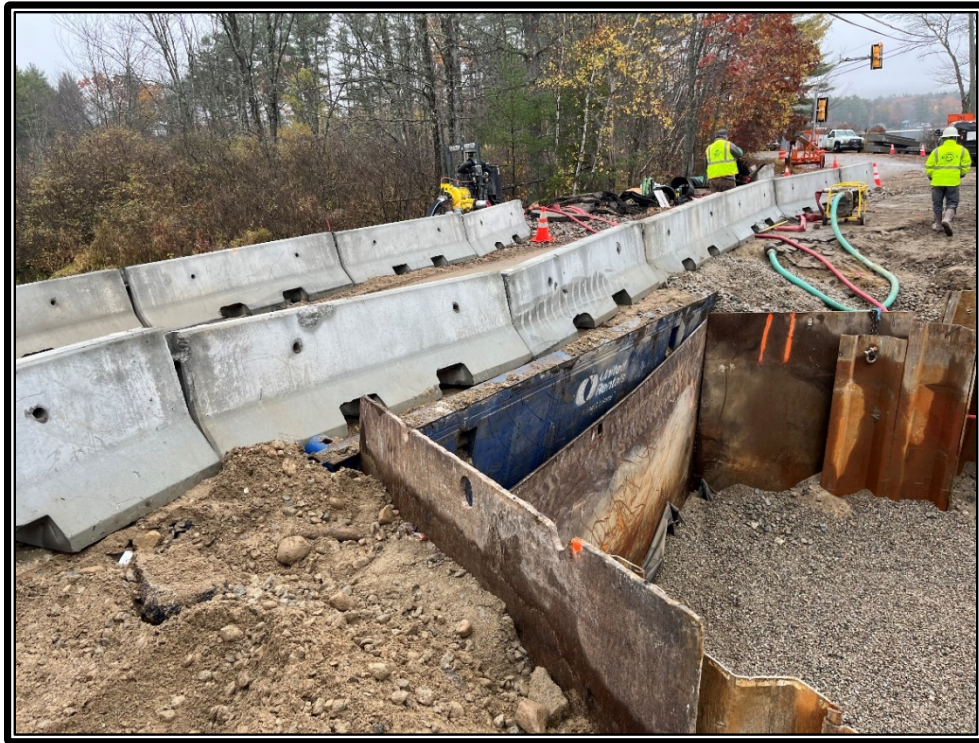
Photo 2: Trench box wall supporting existing roadway.
