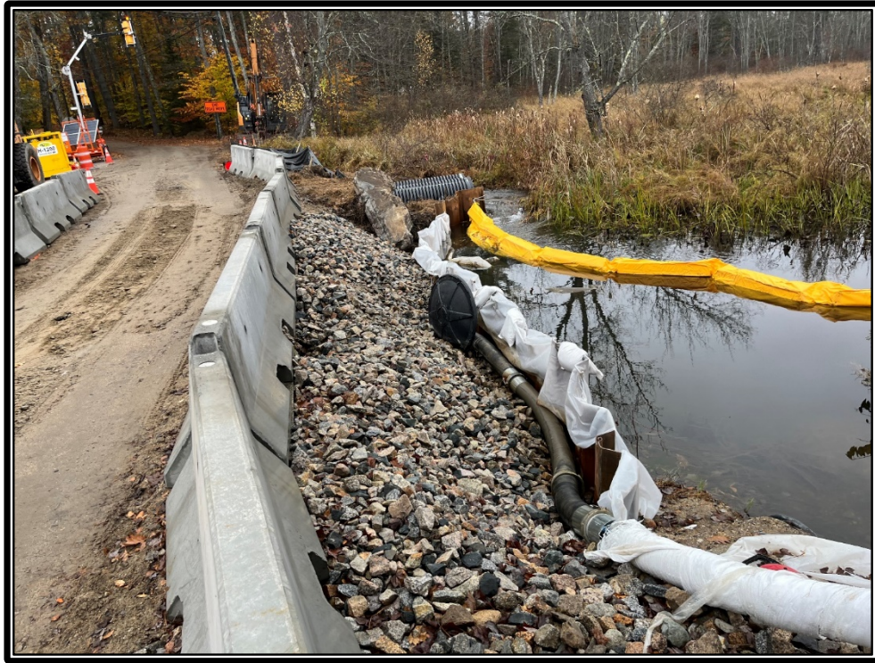
Photo 4: Hole forming along the top of riprap.
