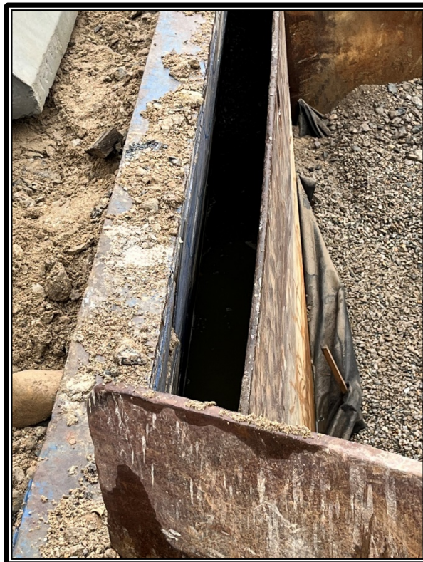
Photo 3: Standing water between trench box wall and road plate.
