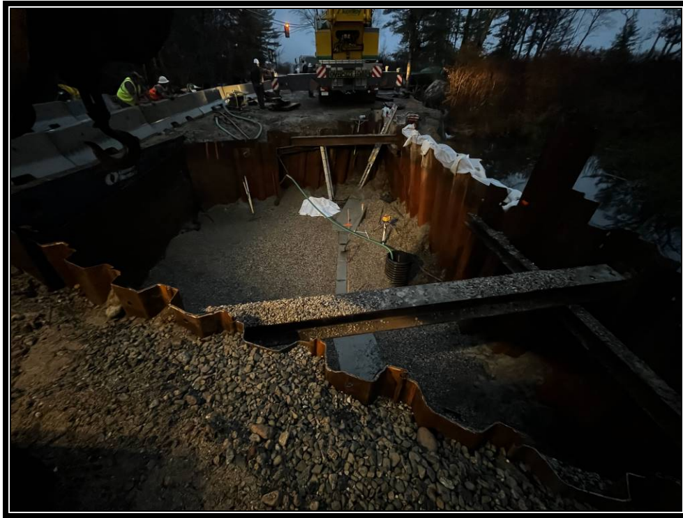
Photo 1: Excavation ready for box culvert installation.
