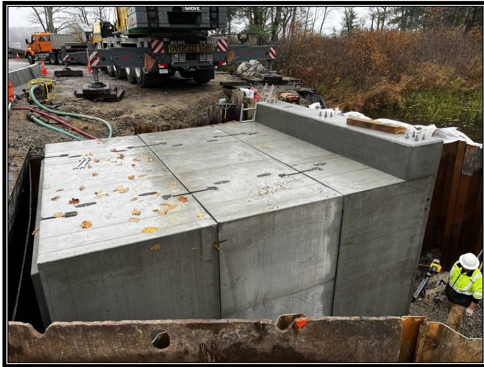
Photo 9: First phase of box culvert installation complete.
