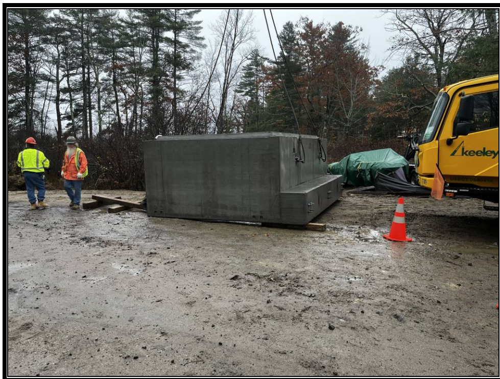
Photo 4: First box culvert segment.
