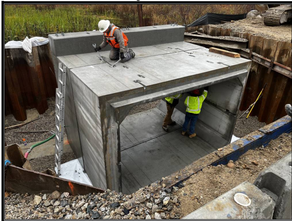
Photo 8: Second box culvert segment in place.
