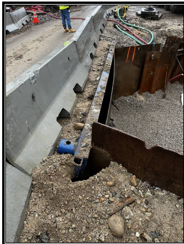
Photo 2: Trench box wall supporting existing roadway.
