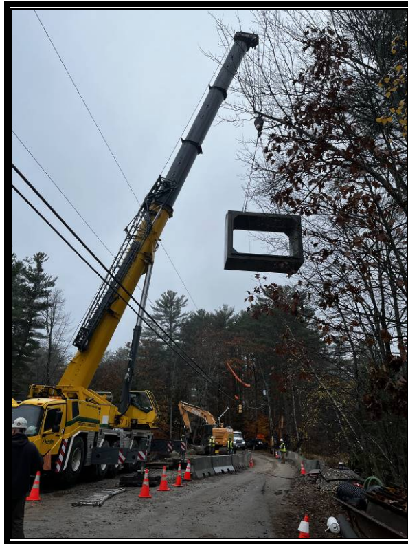
Photo 5: First box culvert segment being craned in.
