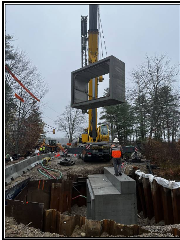
Photo 7: Second box culvert segment being craned in.
