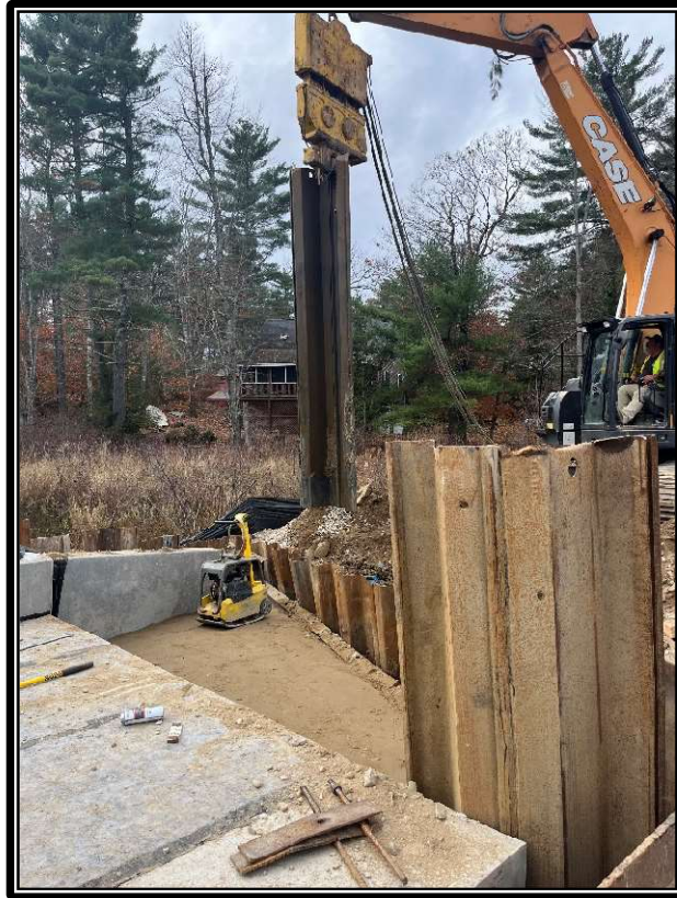
Photo 2: Sheet pile on the sides of the excavation being removed.
