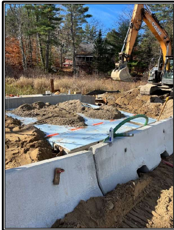
Photo 1: Gravel is placed overtop the box culvert.
