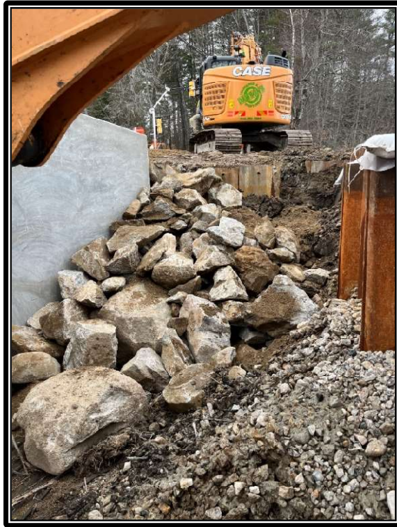
Photo 3: Riprap placed on the northwest corner of the streambed bank reconstruction.
