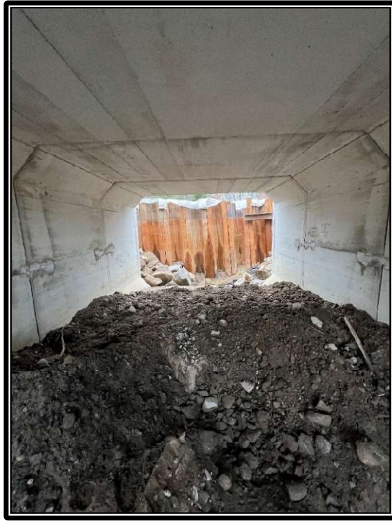
Photo 2: Streambed material was placed through the entirety of the culvert.
