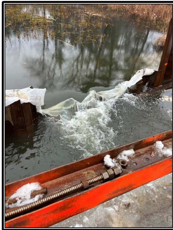
Photo 1: Sheet pile lowered to allow flow through the culvert.
