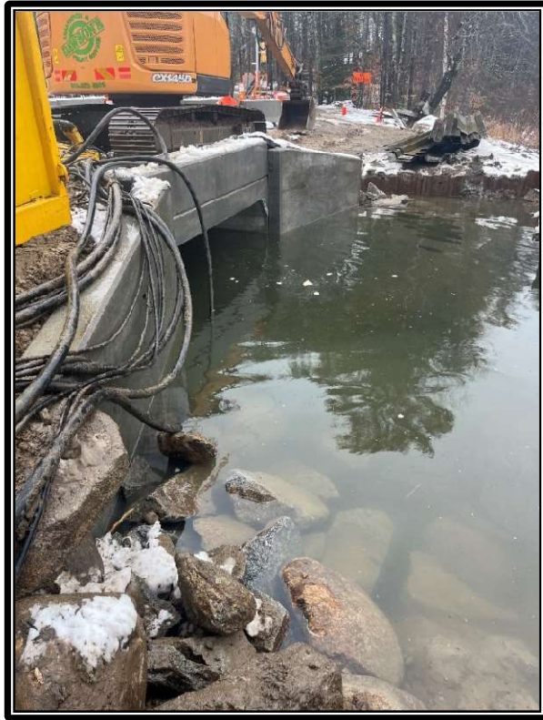
Photo 2: All sheet pile was removed from the channel on the outlet side.
