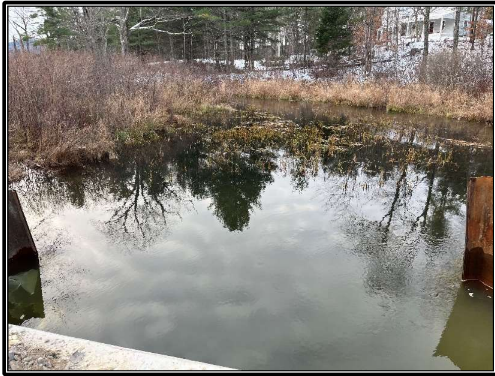
Photo 2: The middle sections of sheet pile were removed from the channel on the inlet side.
