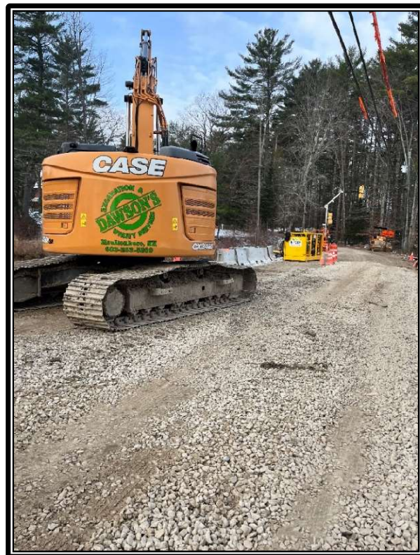
Photo 1: Stone was placed to stabilize the roadway.
